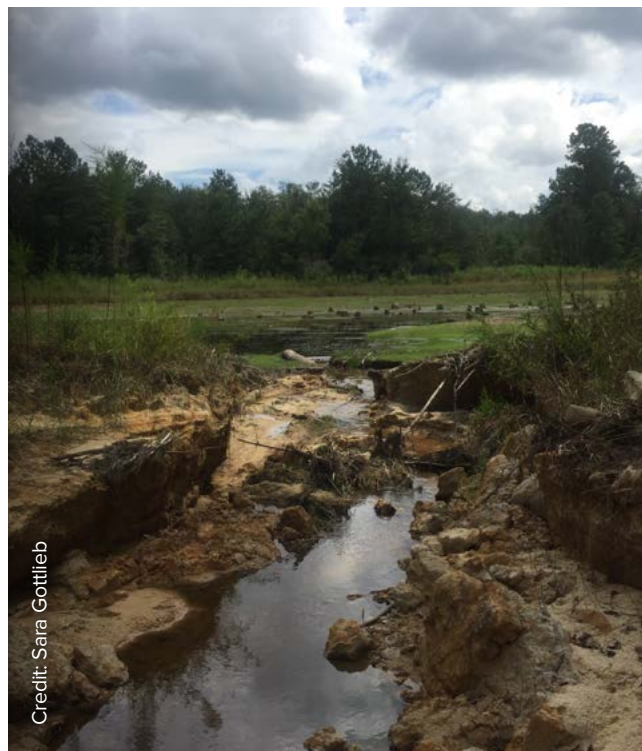
Breach of lowest dam on Hopkins Tract, looking upstream.
