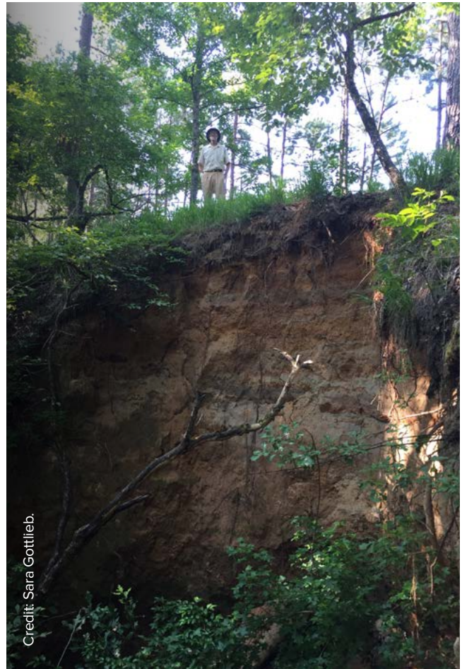
Erosion at Little Pine Knot dam face.
