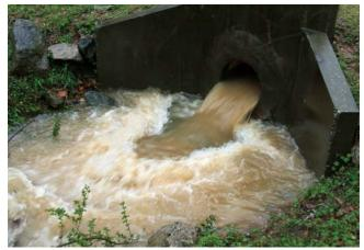
onto the floodplain, or the gradient is steeper in the crossing structure than the channel profile upstream or downstream of the crossing. This increased water velocity can inhibit aquatic and terrestrial wildlife passage, increase the likelihood of scour and erosion, and weaken the structural integrity of crossings. These problems are most likely to occur during high flows and floods, but the signs of scour and erosion may also be evident during low and normal flows.
